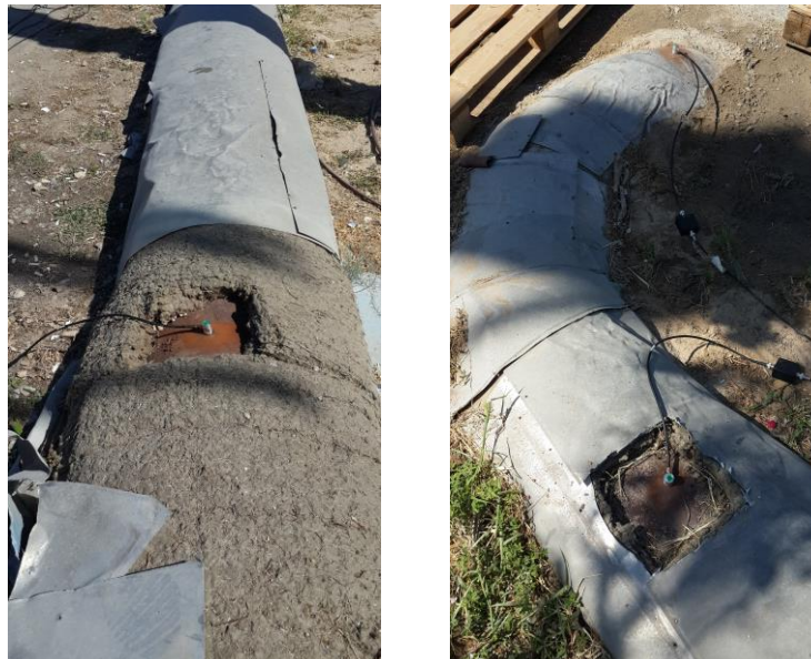
Figure 2. AE sensors installed along insulated piping.
