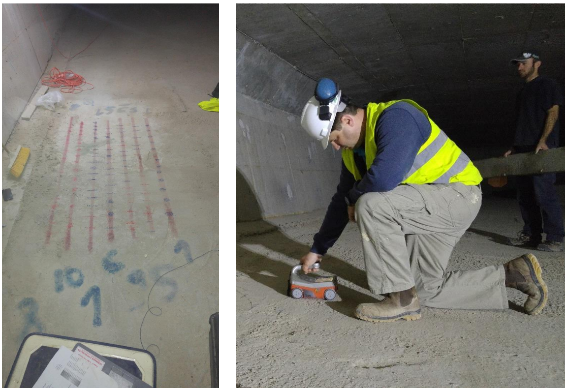
Figure 1. Mapping cable ducts layout using GPR.
